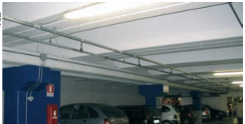
Canalis KBA supplying luminaires nearby sprinklers.
